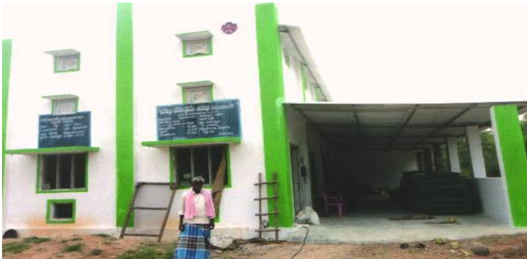
REARING SHED CONSTRUCTED UNDER RKVY WITH VARANDAH
